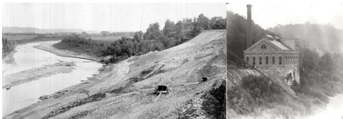
Original Ohio River Intake Construction
